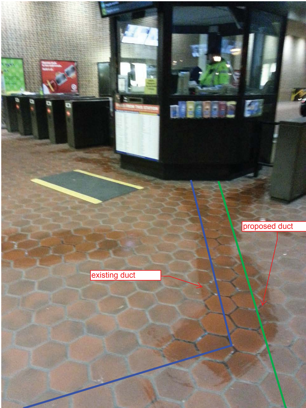
Photo #1 – C13 King Street South: Kiosk with existing and proposed duct runs
